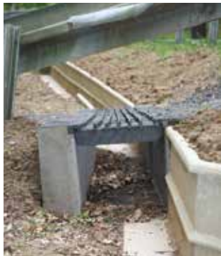
Stop Channel showing alignment with Guide Wall.
